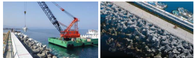
Fig. 1 Block stacking work and the measured point clouds
